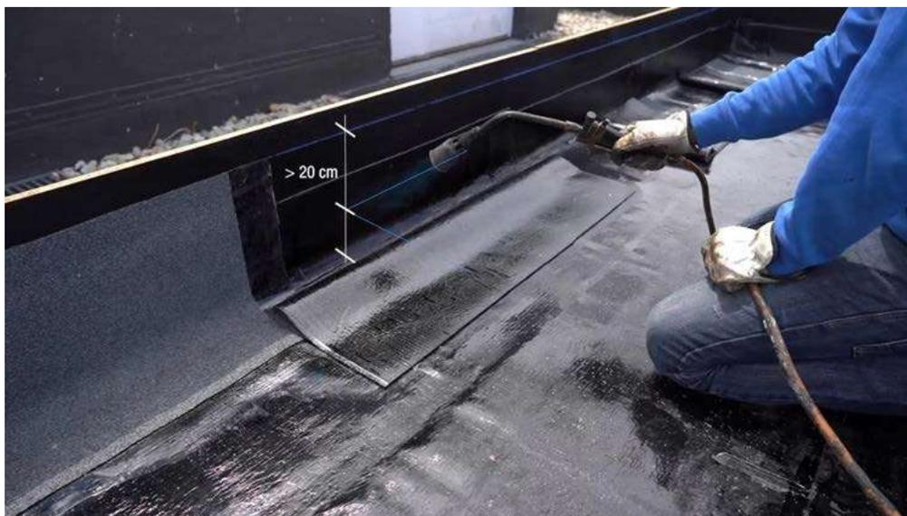
**TIPOLOGÍA DE LÁMINA ASFÁLTICA**
